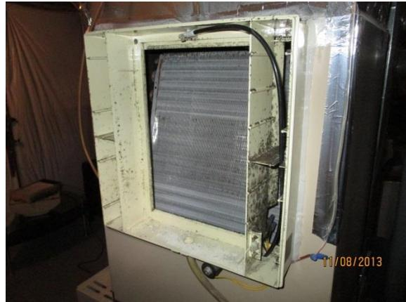
Mold on the HVAC's coil (black area in the middle of the gray metal fins) and the humidifier's plastic frame. This was caused by a faulty humidifier.
