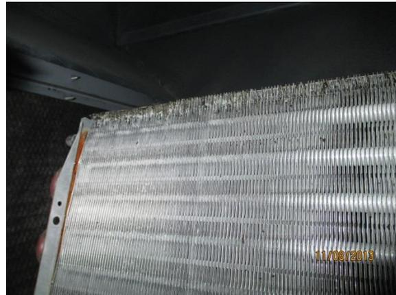
Close up of mold embedded in the fins of this HVAC evaporator coil
