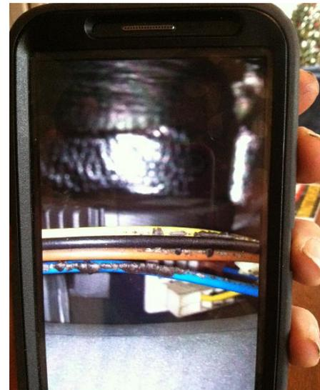
Smudges on wires that an HVAC company tried to pass off as mold
